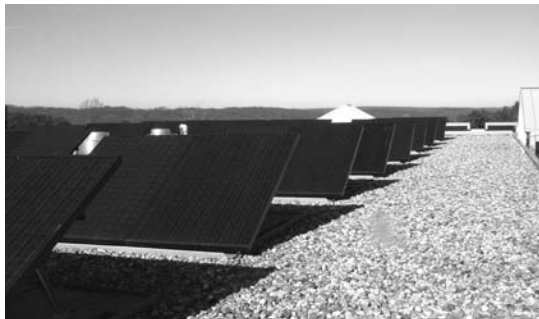
These photovoltaic panels, not visible from the ground, generate electricity atop Park Dormitory in "The Plex." The College Environmental Model Committee is investigating options for adding additional renewable energy generation capacity to the campus.
